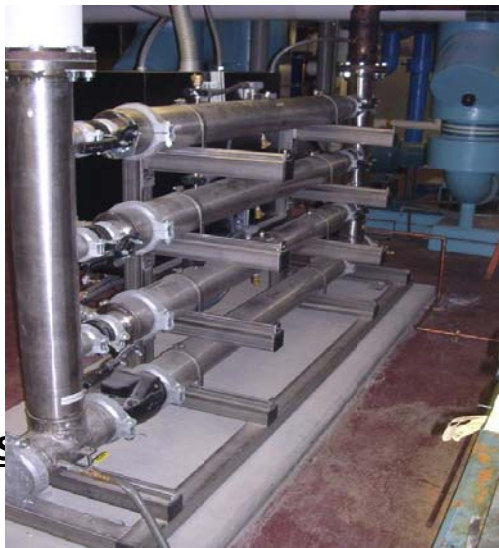
Service arms allow for easy pump inspection. Horizontal Configuration Shown / Vertical Available
