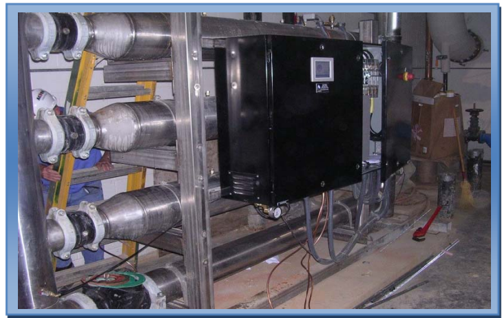
DELTA P Horizontal QuietPak Domestic Water Variable Speed Booster System
